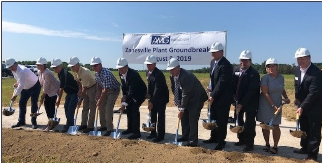
Local officials and company representatives break ground at the AMG Vanadium site.
