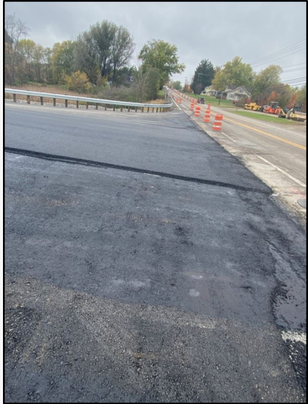
Above: The access road has officially connected with US 40.
