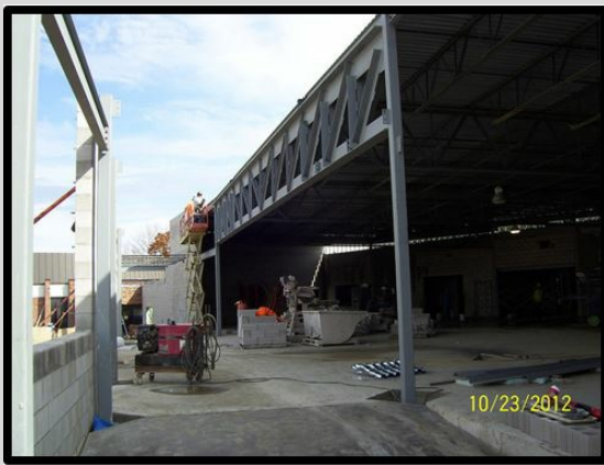
Mideast Career and Technology Center Steel Building
